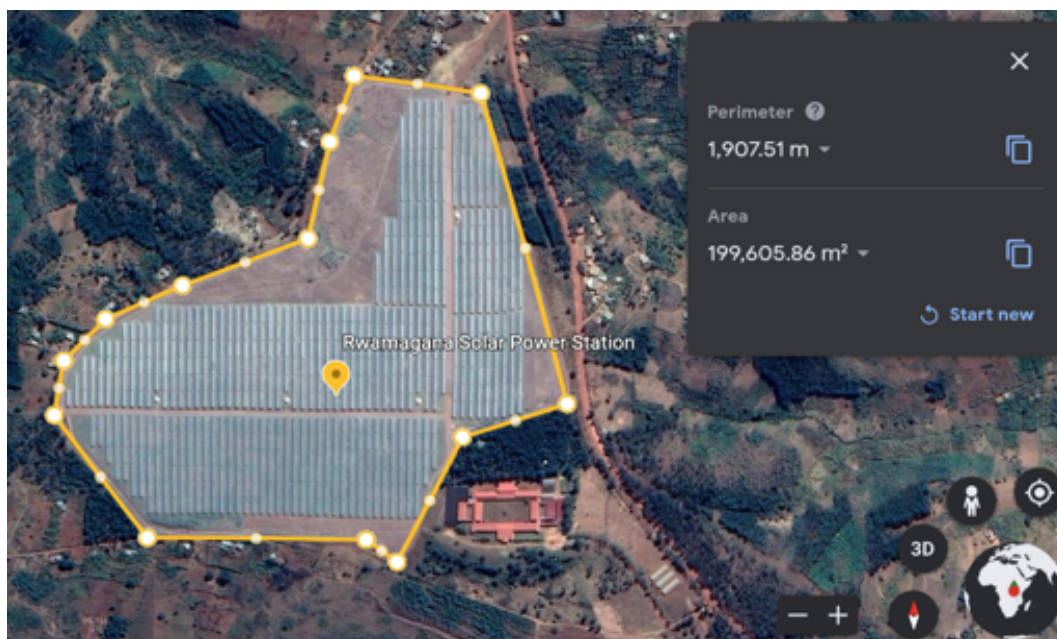
Figure 3.C.2.a-2 Perimeter and Area of the Rwamagana Power Plant
