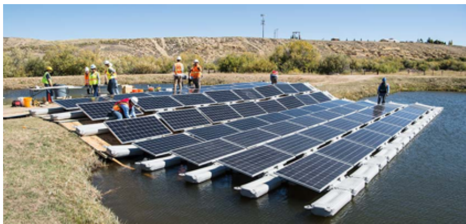
Figure 3.C.2.c-1. Example FPV System being Installed in the US 47
