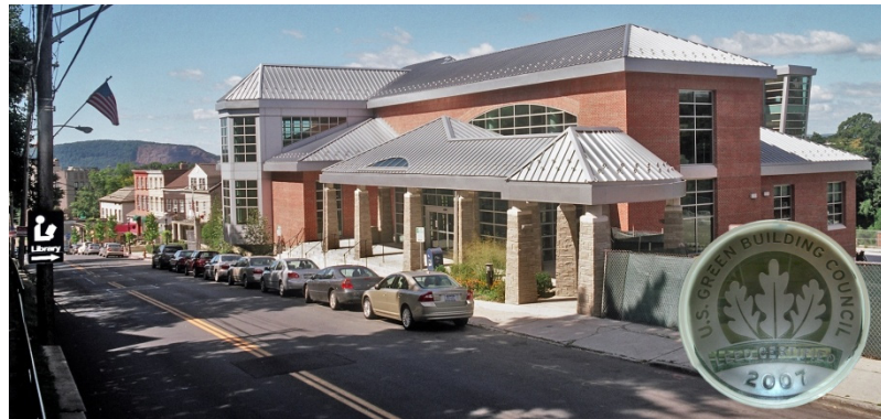
The village and town of Ossining, both Climate Smart Communities, serve residents with a new library, the state's first public building to meet the Leadership in Energy and Environmental Design (LEED) standard. (Photo courtesy of Amiaga Photo, Inc)
