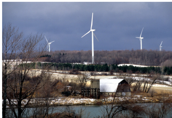
Wind power is an important and growing source of low-carbon electric power. The Fenner Wind Power Facility, located in Madison County, New York, generates 89 million kilowatt hours of electricity each year.
