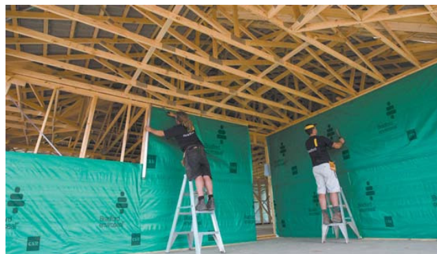
Weatherizing buildings reduces building heating/cooling needs and GHG emissions, and also provides employment to local workers.
